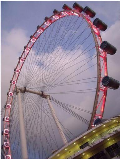
pods) attached to the rim in such a way that as the wheel turns, they are kept upright, usually by gravity.
